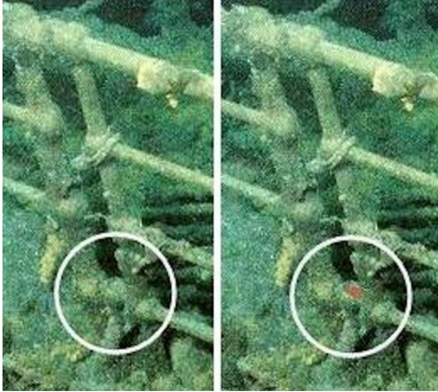
Removable railing connection
