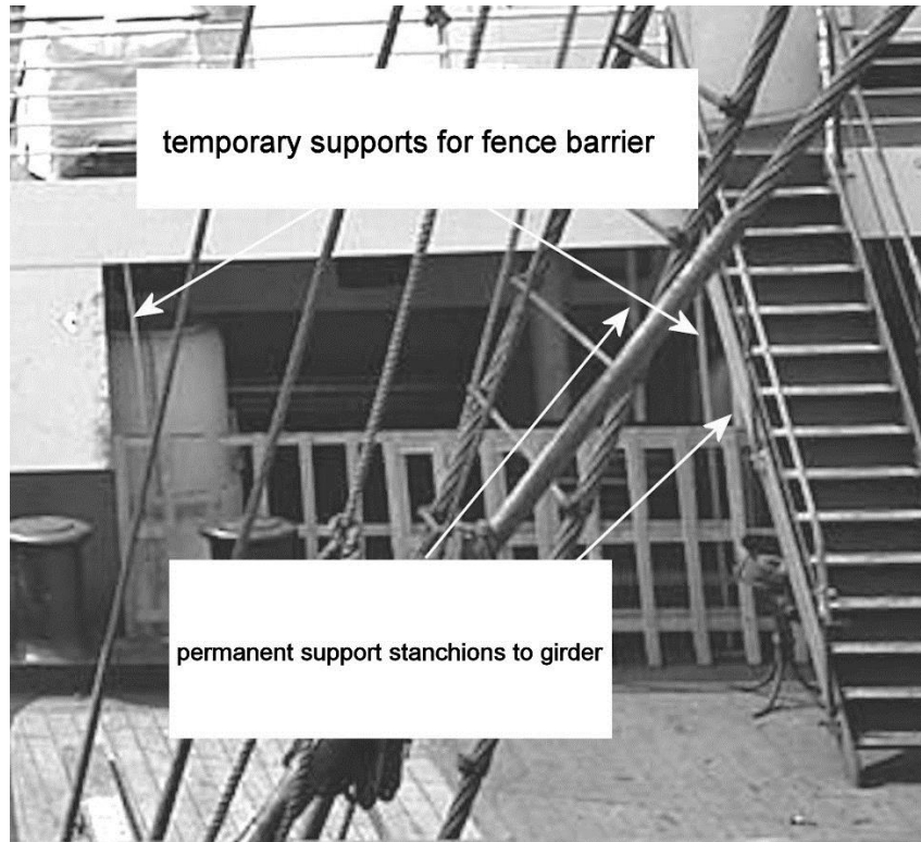
Permanent support stanchions to poop deck girder
